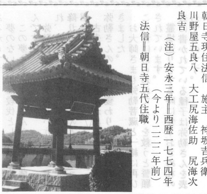
Photograph of the Bell Tower (鐘楼堂) under restoration.
